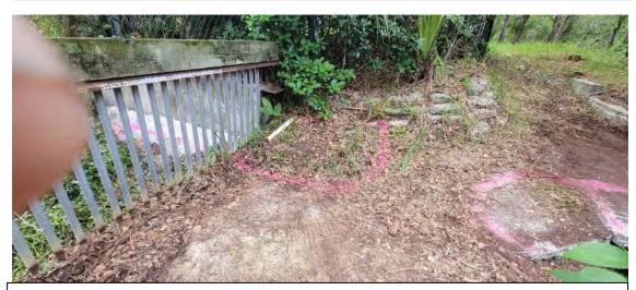
Painted Boundaries (in pink) of Suspected Area of Damaged Concrete Slab in Southwest Corner of Area 2
