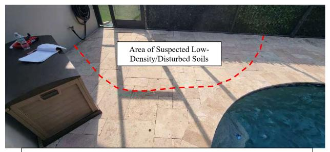
Approximate Boundaries of Suspected Area of Low-Density/Disturbed Soils Under Pool Deck in Area 3
