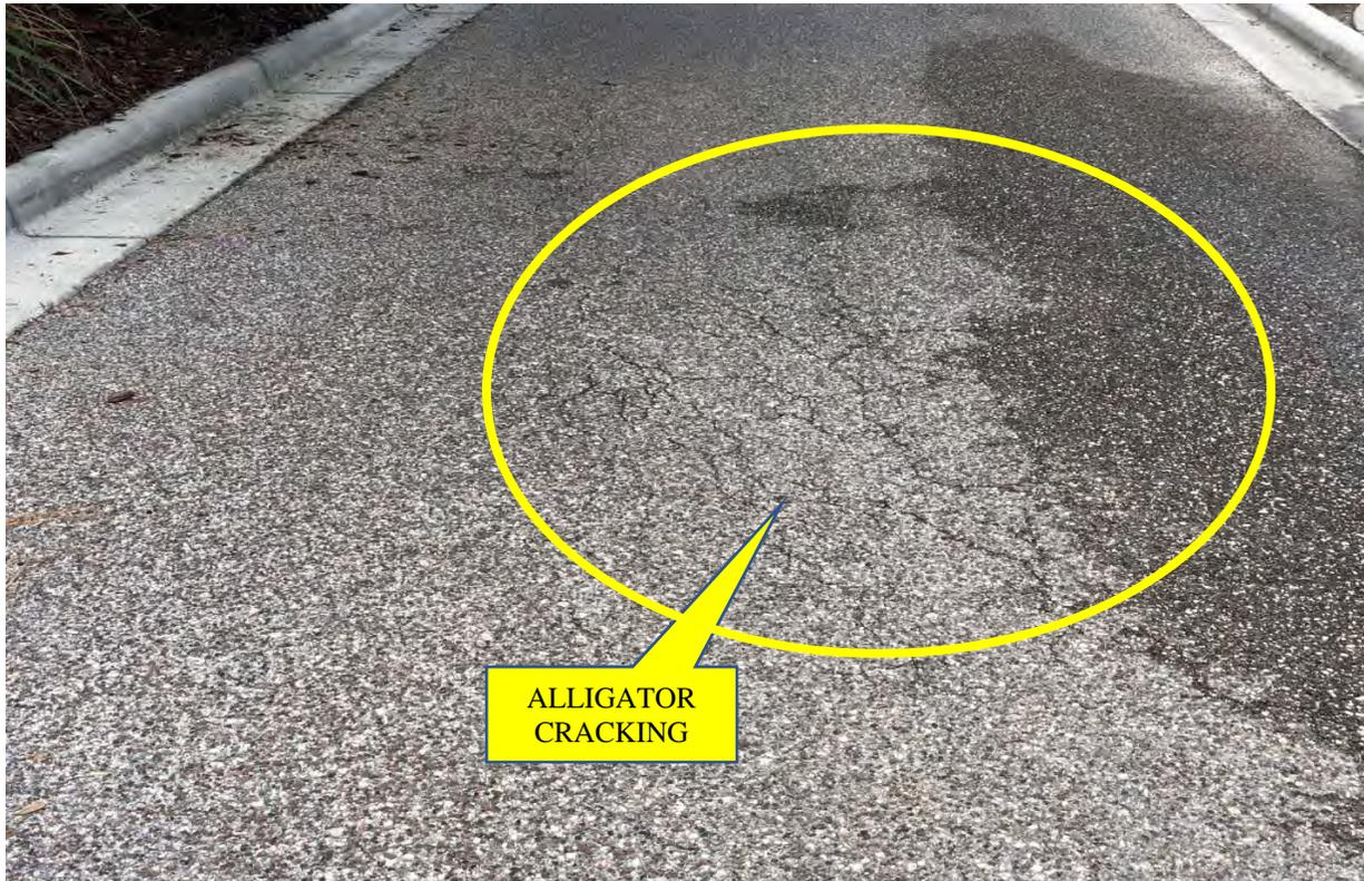
The photo above shows the alligator cracking but the extent is not entirely visible in the photo. The cracking extends most of the way across the pavement width on Splendid Lane south of Canopy Drive (approx. 20 to 30 feet).
